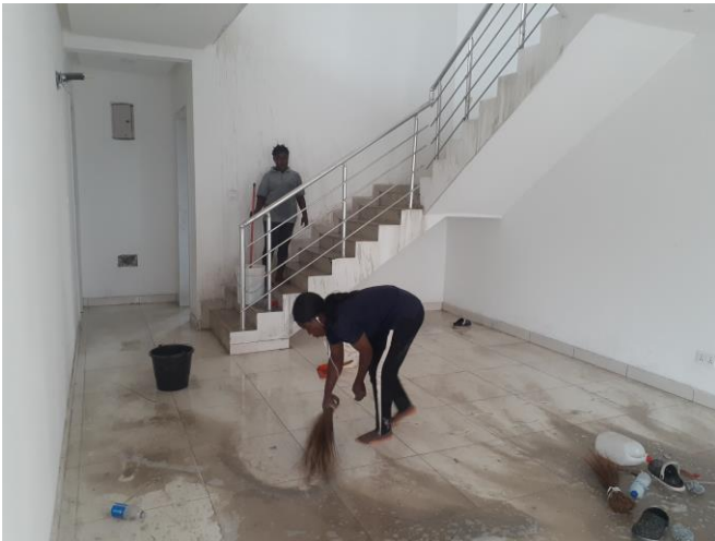
Cleaning was in progress, some stains are found on walls, calls for repainting
