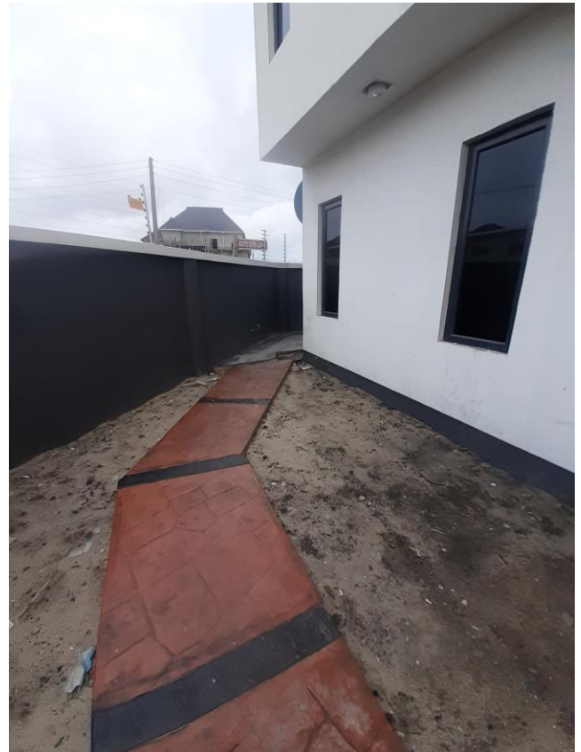
Walkway on the side of the building where landscaping need to be done.
